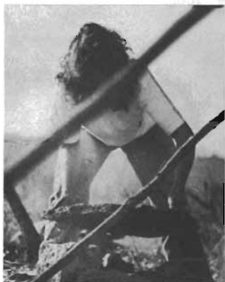
Geri places a flat rock on chimney as rain cap ( above ).
