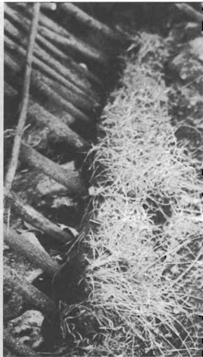
Sod is placed onto the bottom of the south rafters to add to the water-diversion berm (right).
